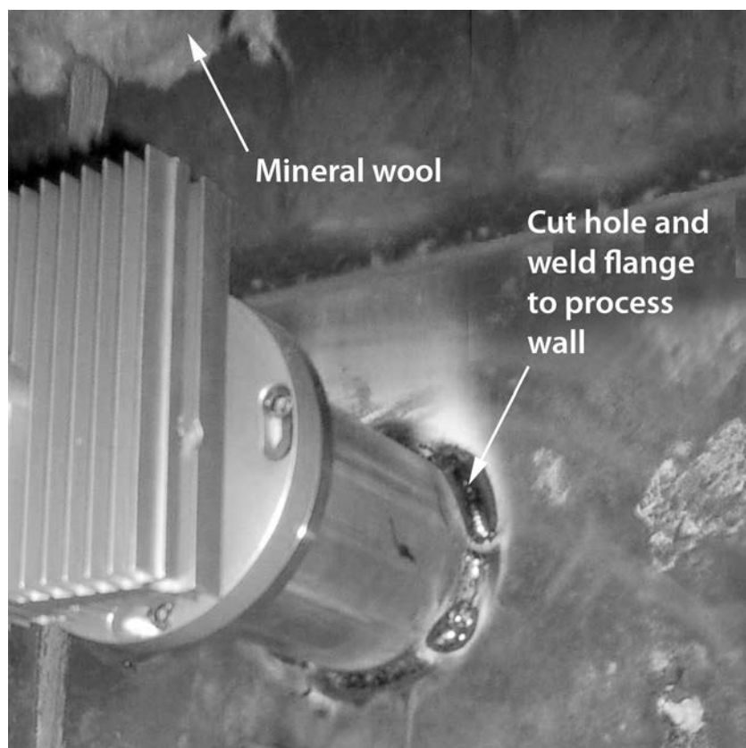
Figure 82 Cooling Set Installation
